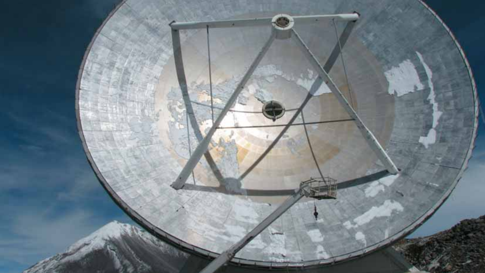
Radiotelescope mirror made by 5M precise sandwich panels
